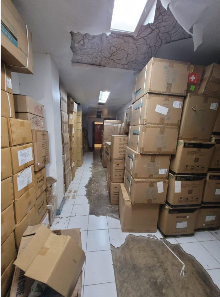
Picture 1: Due to limited space, some supplies were stacked up at the walkway area that leads to the storage room.
